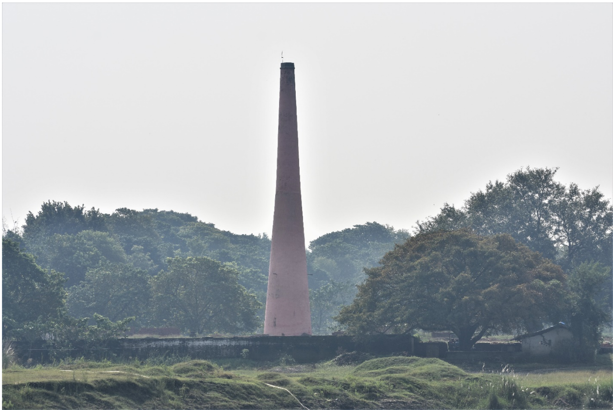
Image 34 : A Brick Kiln As Seen During The Field Survey
