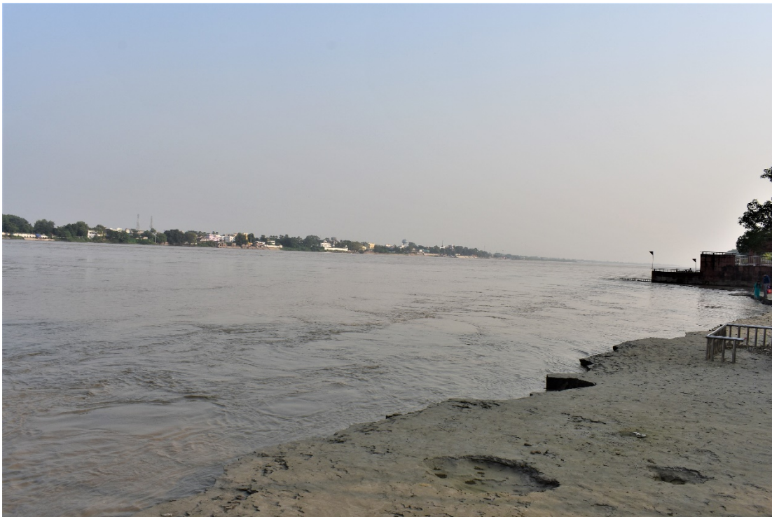
Image 31 : Erosion Prone Bank Along Gandak River As Observed In Sonapur
